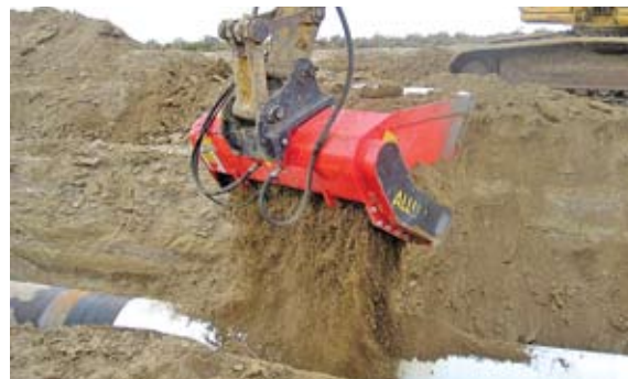
6. Screening of aggregate back into the pipe ditch speeds up the filling process.
