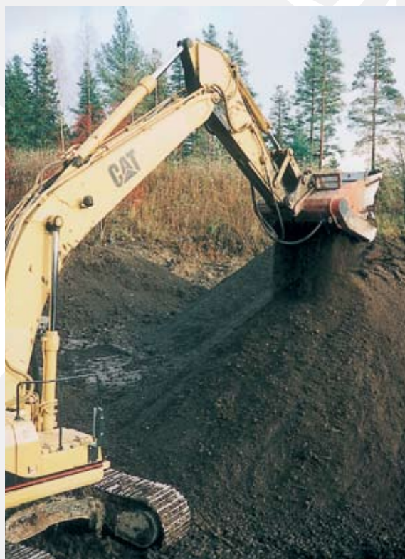
10. Stabilization of clay and contaminated soil.
