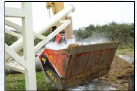
Stabilising soil with lime
